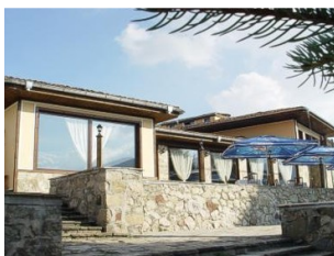
Hotel Kozlekov - restaurant terrace
